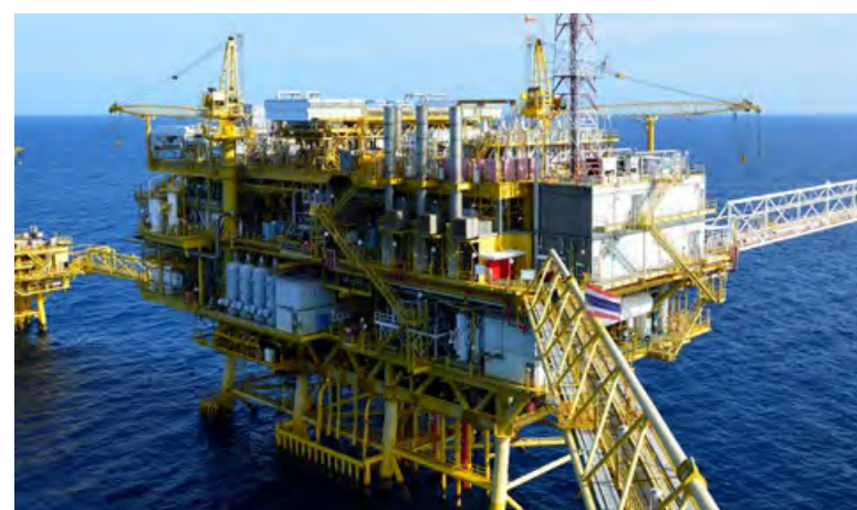
With the acquisition of offshore specialists SAS in England, BAUER successfully expanded its activities in the oil and gas sector.
