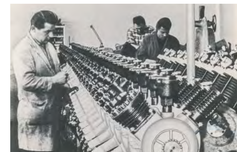
A block assembly line at the plant in Wolfratshausen Strasse.
