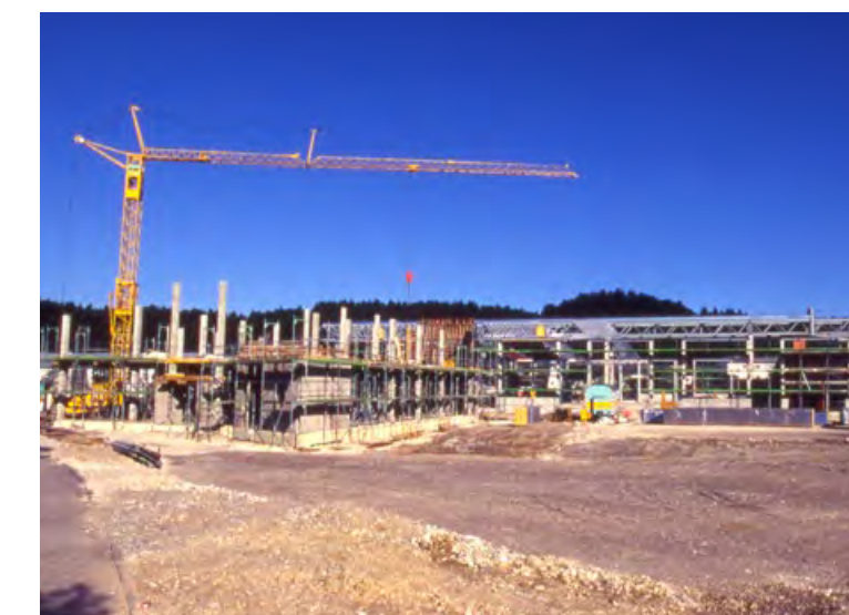
With the new UNICCOMP component plant south of Munich, BAUER at a stroke doubled its production capacity.
