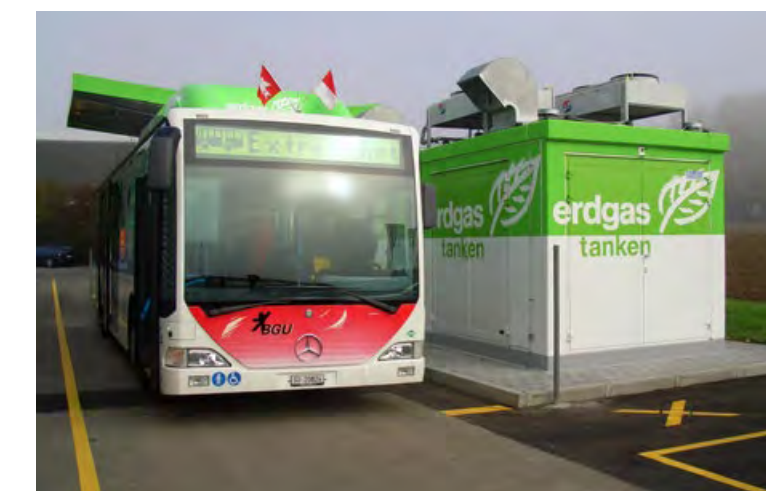
A BAUER natural-gas filling station for bus refuelling on the premises of the public utility company in the Swiss town of Grenchen.
