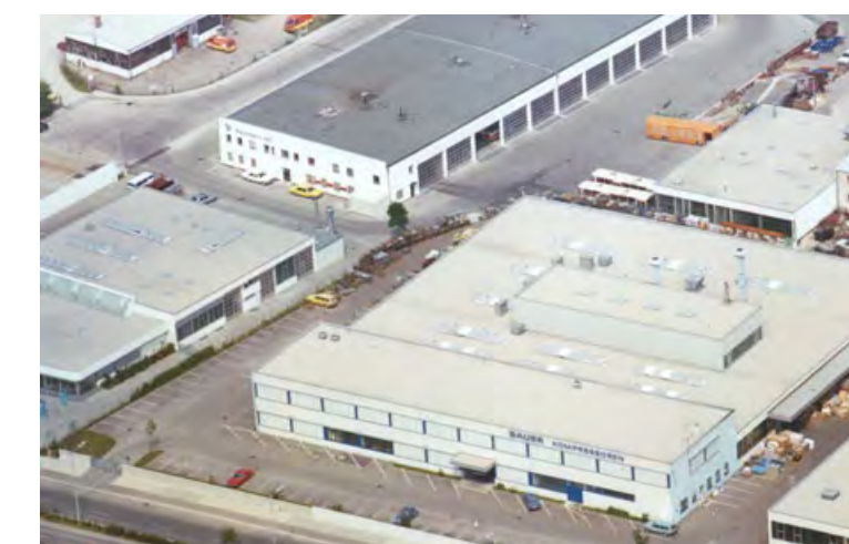
A bird's-eye view of BAUER's completed plant in Drygalski-Allee
