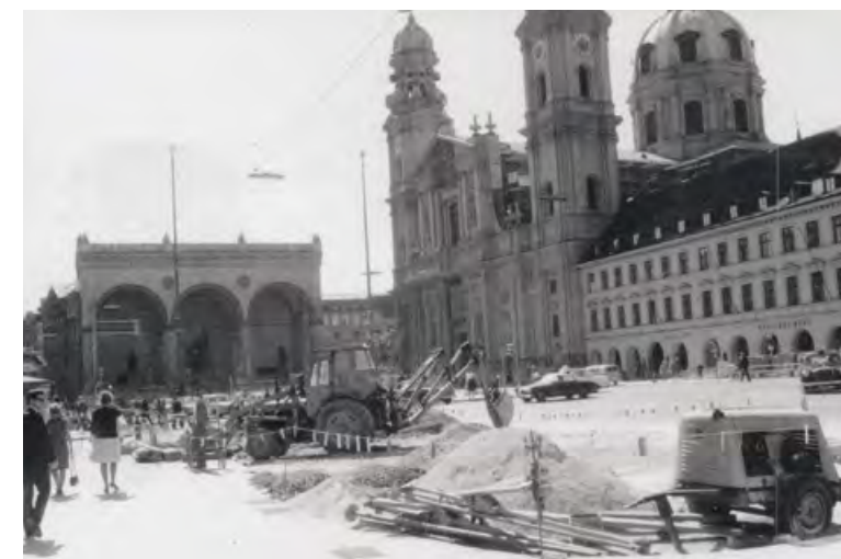
This is what Munich looked like after the War – with the first BAUER compressor used for the clearing work.
